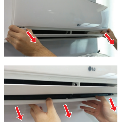
Figure 42: Removing the Bottom Cover, Alternate View.
