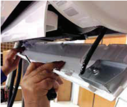
Figure 89: Reattaching the Bottom Panel.
