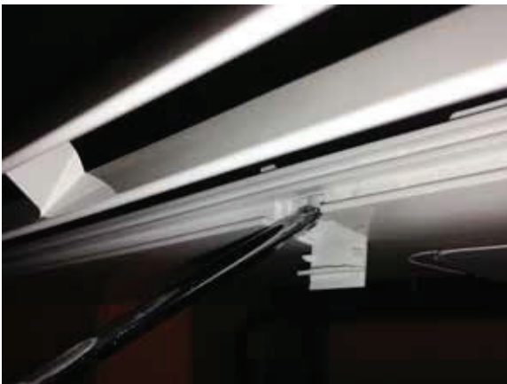
Figure 15: Remove Screws from Bottom Panel.
