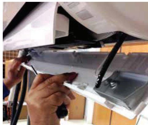
Figure 73: Remove Bottom Panel.
