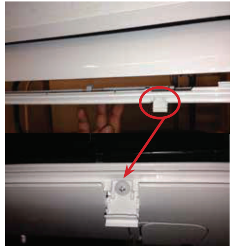
Figure 91: Reattaching the Screws on the Bottom Panel.
