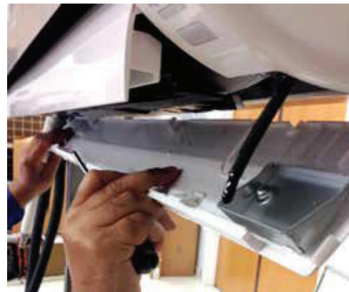
Figure 16: Remove Bottom Panel.
