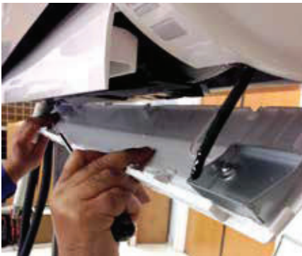
Figure 89: Reattaching the Bottom Panel.
