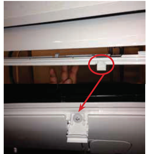
Figure 91: Reattaching the Screws on the Bottom Panel.
