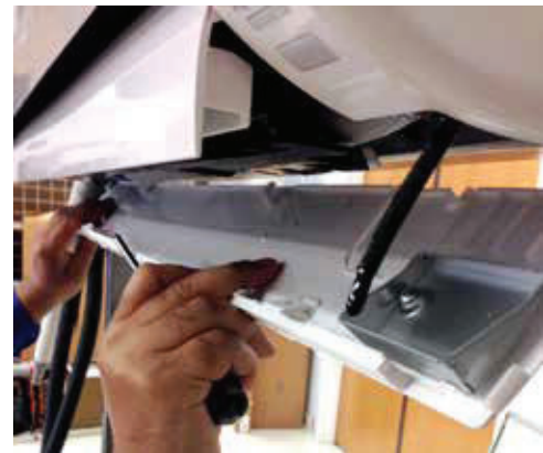
Figure 16: Remove Bottom Panel.
