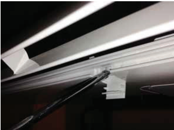
Figure 72: Remove Screws from Bottom Panel.
