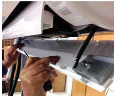
Figure 73: Remove Bottom Panel.
