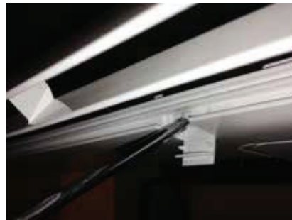
Figure 90: Reattaching the Screws on the Bottom Panel.
