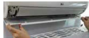
Figure 94: Securing the Bottom Cover C-hooks to the Indoor Unit Sockets (Step 3).
