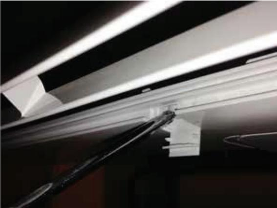
Figure 14: Latch over Screws on Indoor Unit Bottom Panel.
