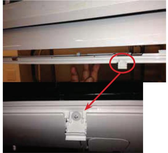
Figure 15: Remove Screws from Bottom Panel.
