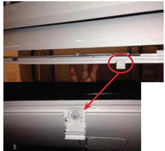
Figure 72: Remove Screws from Bottom Panel.
