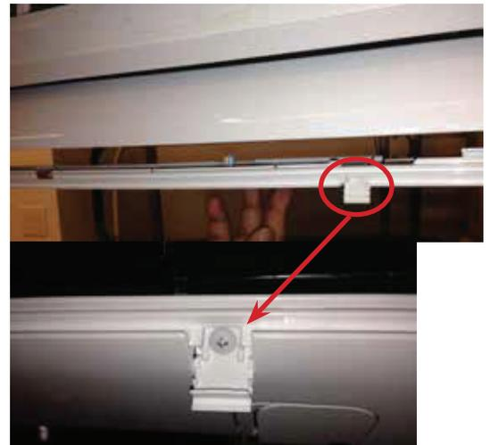
Figure 72: Remove Screws from Bottom Panel.
