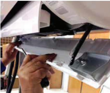
Figure 90: Reattaching the Screws on the Bottom Panel.
