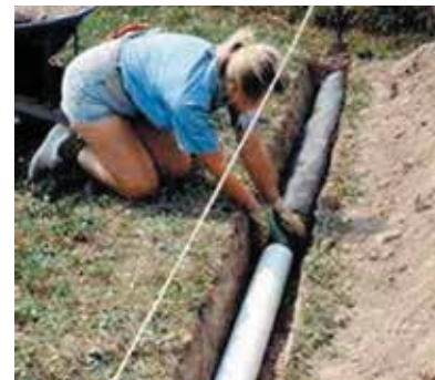
Figure 65: Underground Refrigerant Piping.
