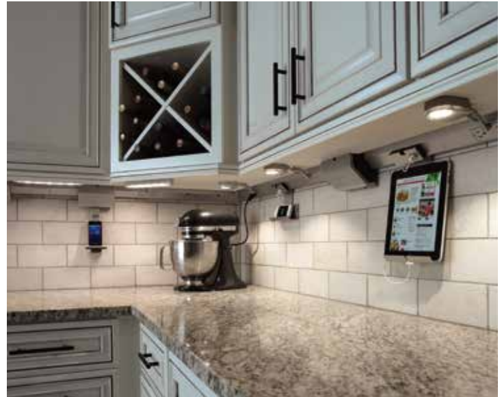
Under-Cabinet Lighting System installed in a kitchen.
