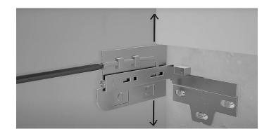
The top screw adjusts the vanity up and down, and the bottom screw adjusts the vanity front to back.
