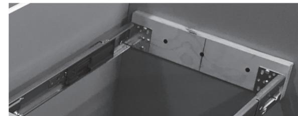
3. Line the front of the slide up with the edge of the face frame. Using the front hole of the cabinet member, predrill a hole using a 1/8" drill bit. Secure each cabinet member to the face frame of the cabinet using one #6 x 1/2" screw (included) per side.
