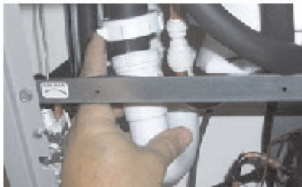
Reattach drain line to P-trap
