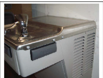
Remove Basin Fasteners
