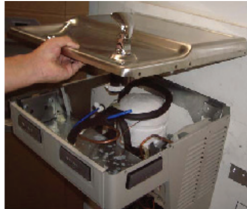
Lift and Remove Basin.
