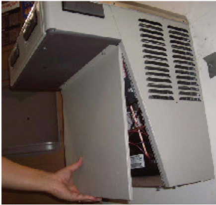
Remove Front Panel
