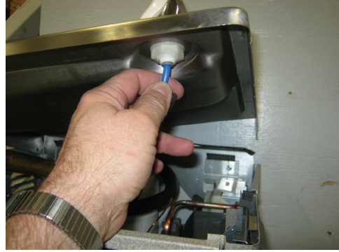
Remove Bubbler Water Line
