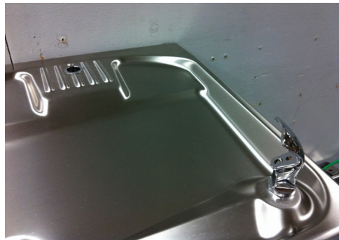
Exchange Bubbler hardware.
