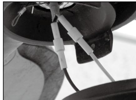
3. Connect white-to-white and blue-to-black wires.
