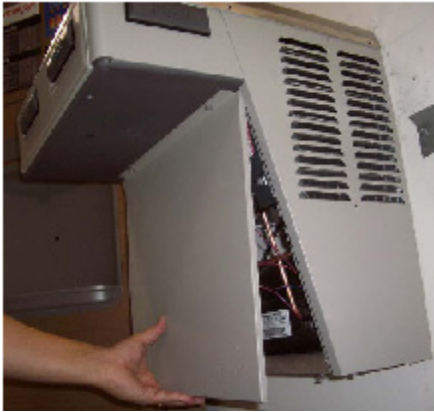
Remove Front Panel
