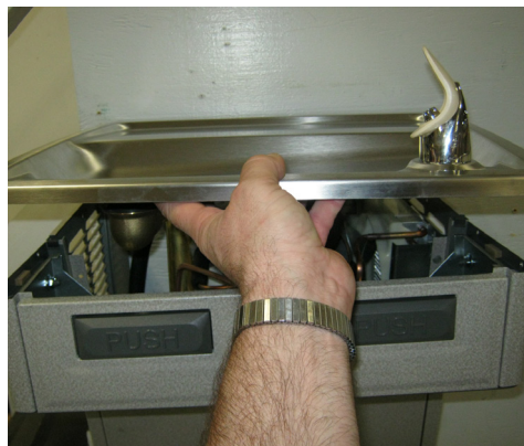
Lift and Remove Basin.
