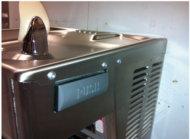
Fasten Basin Assembly in place.
