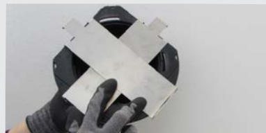
F1-1. Place two SUPACLPB clips perpendicular to each other under the pedestal base.
