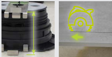
E3-4. Cut the tile. The dimension of the tile is equal to the distance between the SUPACL PT clip and the SUPACL PB clip.
