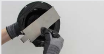
E3-1. Place the SUPACL PB clip under the pedestal base.
