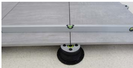
16. Check to make sure that the flooring is leveled.
