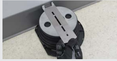
D2-2. Place the SUPACLPP spacer clip on the head of the pedestal.
