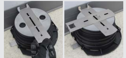
D3-3. Place SUPACL PP spacer clip perpendicular. Place SUPACL PT.
