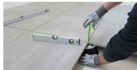
17. If it is not leveled, adjust the height with the SUPAK tool.
