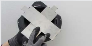
F3-1. Place two SUPACL PB base clips perpendicular to each other under the pedestal base.
