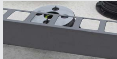
E2-2. Place the BSR profile between the tabs on the head of the pedestal.
