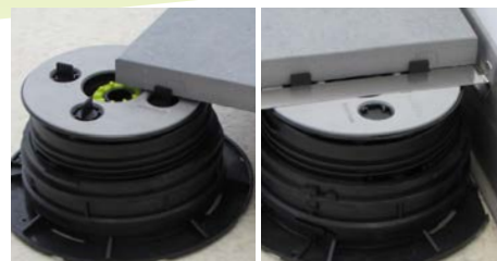
14. Place the corners of the tile between the tabs.
