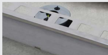
E1-5. Wedge the cut tile between the BSJ profile and the SUPACLPB clip.
