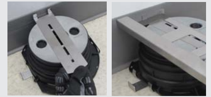
D1-3. Place the SUPACLPP spacer clip and the BSJ profile on the head of the pedestal.
