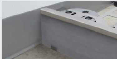
D1-5. Wedge the cut tile between the BSJ profile and the SUPACLPB clip.
