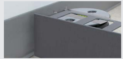
D2-2. Place BSR profile on the clip on the head of the pedestal.
