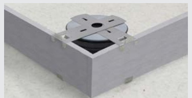
F3-5. Wedge the cut tile between the SUPACL PT clip and the SUPACL PB clip.
