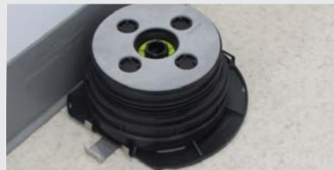
D3-2. Place the pedestal with one cut side against the wall and the other facing outwards.
