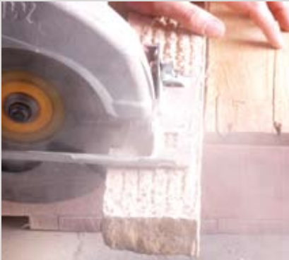
Trim stones to fit Option A - circular saw
