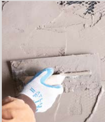
Apply mortar setting bed
