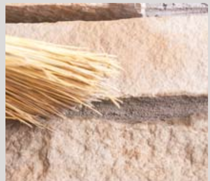
Brush off excess mortar with a dry brush
