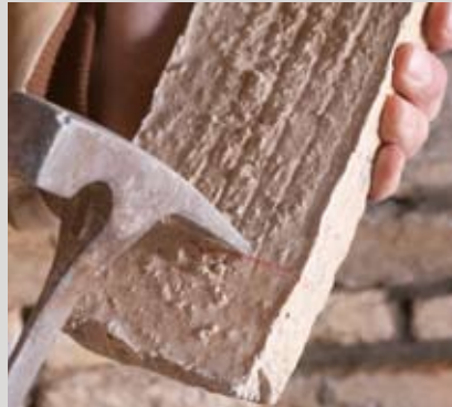
Trim stones to fit Option B - hammer
