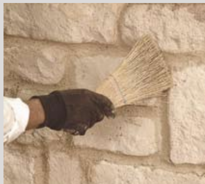
Brush off excess mortar with a dry brush
