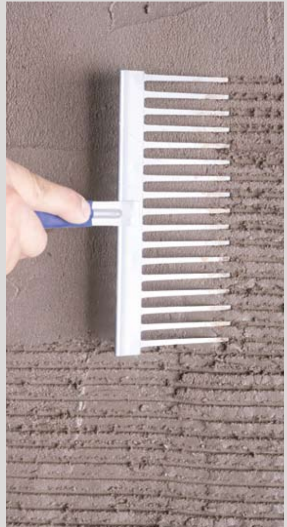
Rake mortar setting bed
