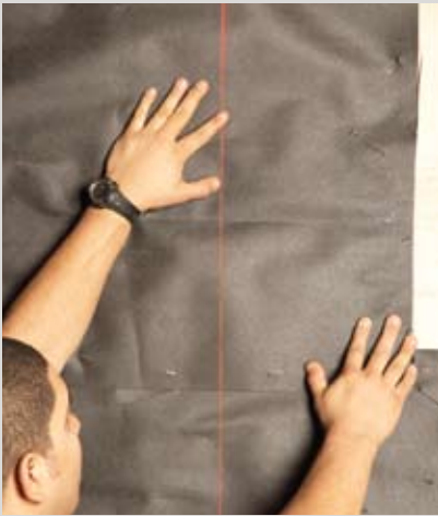
Install Water Resistant Barriers (exterior applications)
