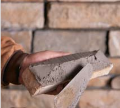
Apply mortar to the entire back of stone
