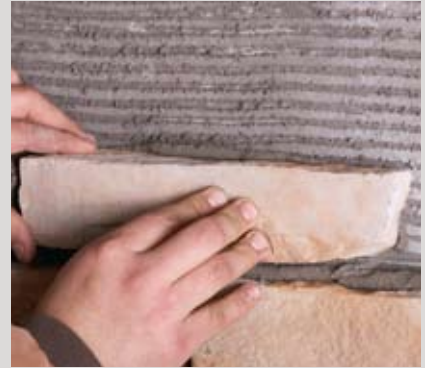
Install flat stones
