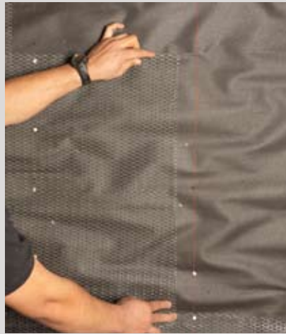
Install corrosion resistant metal lath
