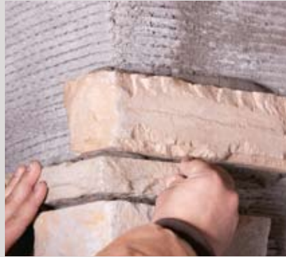
Install corner stones first
