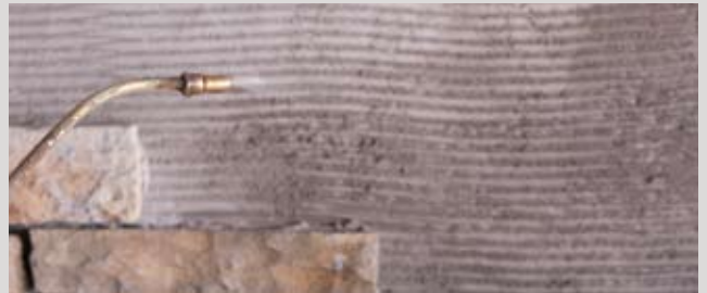
Moisten the scratch coat and the back of the Stone, especially in hot or windy climates
