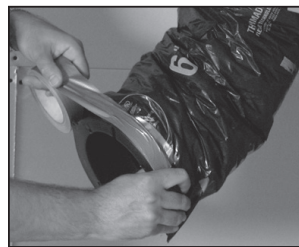
Figure 9 Finish by taping the vapor barrier to the collar to ensure proper seal.
