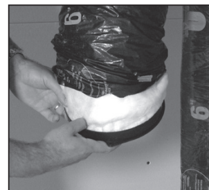
Figure 8 Insert insulation inside the double collar.
