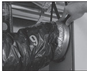
Figure 10 Slide collar into the keeper section of the unit.
