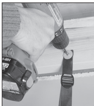
Figure 5 Attach the adjustable hanging straps to the floor joist with four, #10x1" screws. The screws are inserted through one of the links in the hanging chains.
