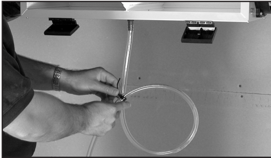
Figure 12 Create a trap by forming a loop in the condensate tubing. Ensure this trap will not be exposed to temperatures where the condensate can freeze.
