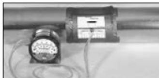
Seal airflow gride in duct with duct tape
