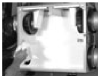
4. Wash out the walls of the unit.
