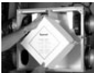
2. Slide out the energy core.
