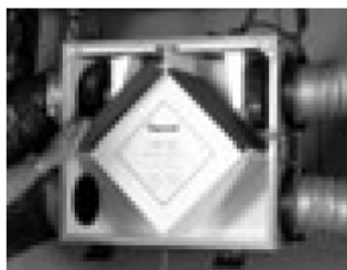
1. Slide out the filters.
