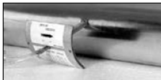
Inserting airflow grid in duct
