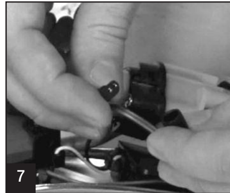
7 Join module connections and secure wiring into integrated clamp.
