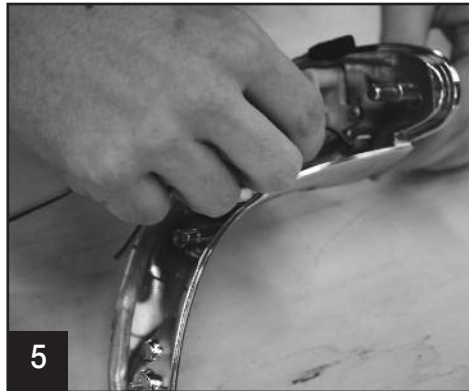
5 Prepare to install new module. Feed green battery wire through hole in faucet base, insert green adapter.
