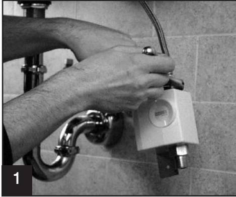
1 Connect SSPS unit. Attached to faucet and install water supply line.
