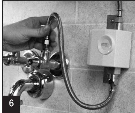
6 Attach to supply. Attach inlet hose to supply and turn on water. With water on, check system for leaks.
