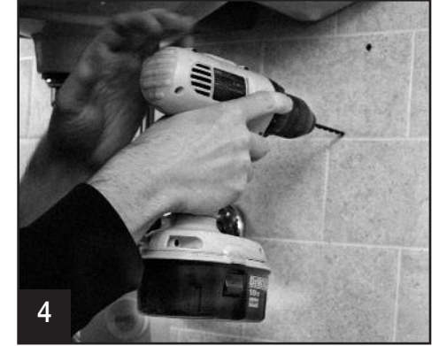
4 Drill holes. Drill holes for screw anchors.
