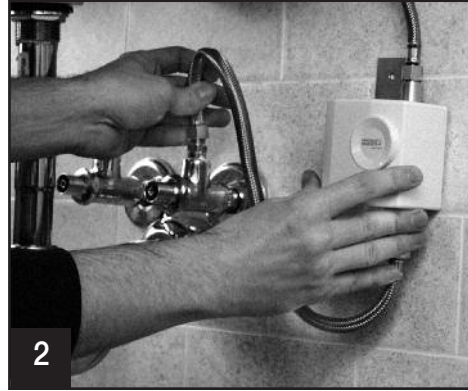
2 Position SSPS under sink. Carefully position to allow connection of water lines and wiring.
