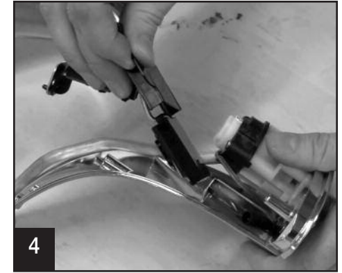
4 Remove electronics module. Carefully remove battery housing and IR sensor. Separate wire connections.
