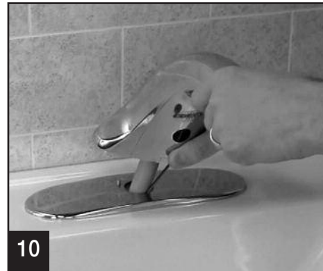
10 Re-install Faucet. Secure faucet to sink.
