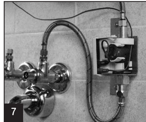
7 Connect wiring. Remove cover and connect faucet wire to SSPS and secure into wire harness.
