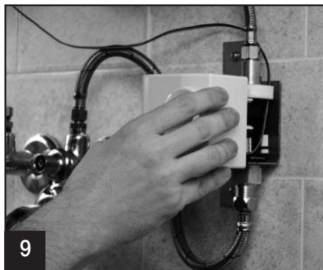
9 Attach cover plate. Faucet will run through programming sequence.
