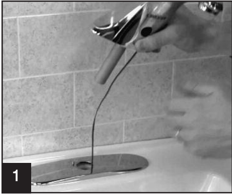
1 Remove the faucet. Turn off water supplies and disconnect power source.
