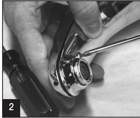
2 Disassemble the faucet. Remove spout to expose faucet body and electronics.
