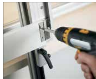
2) Fix back fixing bracket.
