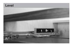
Check to ensure that the runners are level, perpendicular to the face of the cabinet, and parallel to each other.
