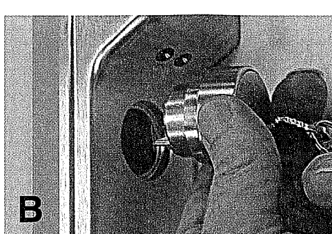
B. Remove old cylinder and Insert new cylinder.
