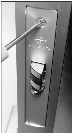
Fig. 7b: Install the latch face plate
