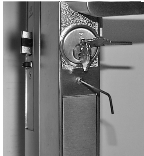
Fig. 12: Turn key counterclockwise and tighten the cover screw.
