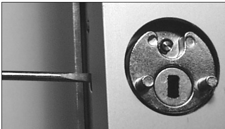
Fig. 7a: Tighten the interface cylinder set screw
