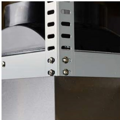
21. Take the inner chimney cover and slide it up flush with the ceiling plate.
