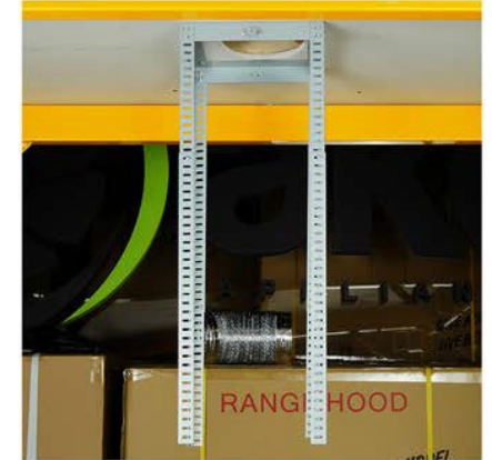
12. The completed support frame will look as pictured.
