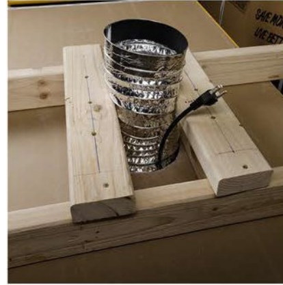
19. Secure the duct to the damper/air flapper with HVAC foil tape (as pictured) or duct tape.
