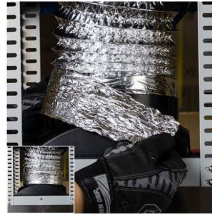
23. Plug in the power cord to the outlet in the ceiling. If no outlet is available, one will need to be installed. The outlet can also be installed outside of the ceiling, but modification to the inner chimney will be required to accommodate the power cord.
