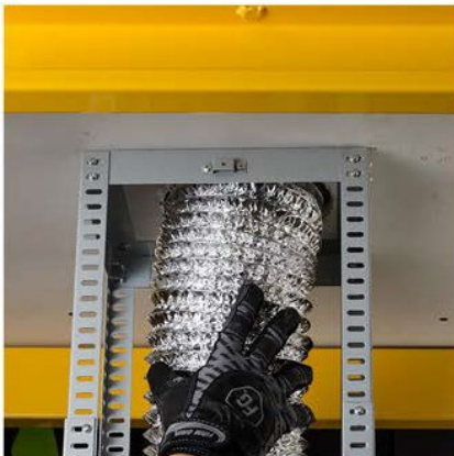
13. Using the included duct pipe, insert it through the hole in the ceiling and connect it to your existing duct work (if applicable). You may need roof access.
