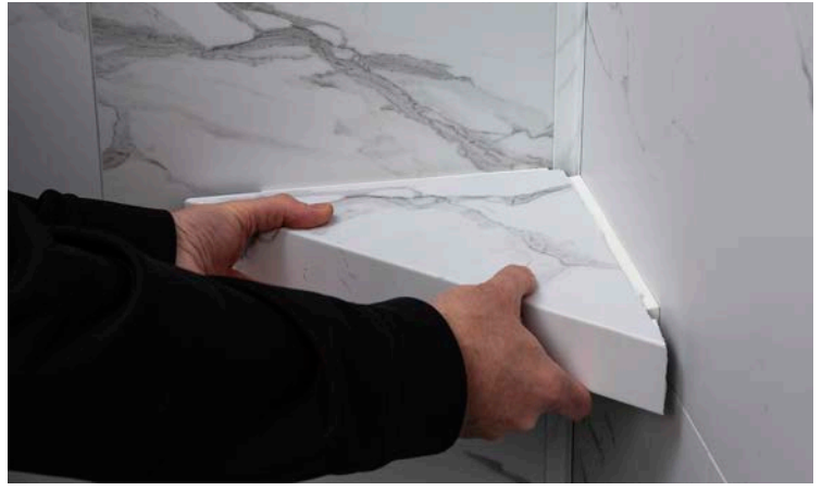
Continue to push the shelf into place for a tight fit against the wall.
