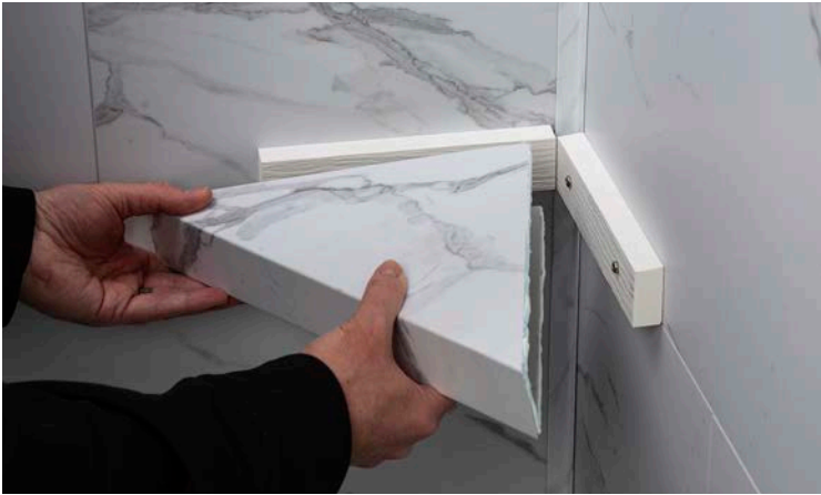
Carefully slide the shelf onto the brackets.
