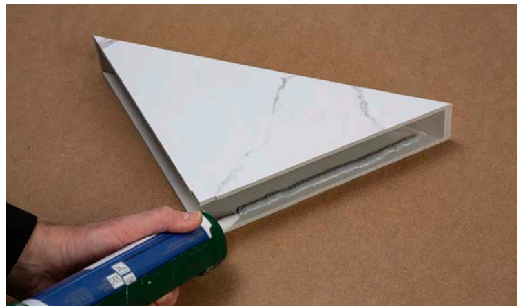
Before installing the shelf, place a bead of adhesive on both inside edges of the shelf. Placing adhesive here will help eliminate glue pushing out onto the outside surfaces of the shelf.
