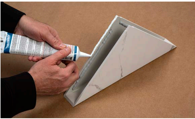
After you have applied the adhesive, place a small bead of sealant along the edges that will go against the shower wall.
