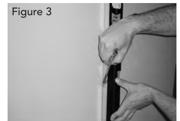
Mark horizontal & vertical reference points
