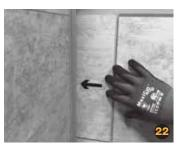
Apply sealant to the interlocking edges if this installation is for a wet environment.
