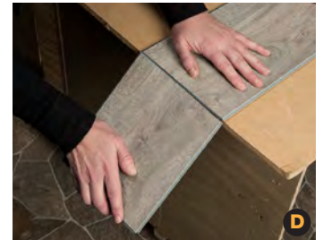
Cut Palisade planks by scoring and snapping with a utility knife. (image C, D). This method may require sanding the snapped edges.
