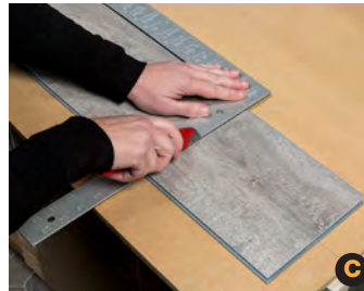
Cut Palisade planks by scoring and snapping with a utility knife. (image C, D). This method may require sanding the snapped edges.
