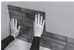
When placing tiles on the second row and beyond, angle the tile back about 30 degrees and rest the bottom edge on the tile below, then slide it over to abut the previous tile.
