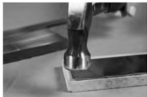
Use a hammer to straighten tile edges. Place the cut tile with the bent edge facing up on a smooth, flat hard surface. Lightly strike the bent edges with the hammer until the edge flattens out.
