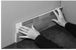
Beginning from inside corner on right, place the first tile.
