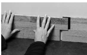
Install next tile as shown.
