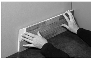
Beginning from inside corner on right, place the first tile.
