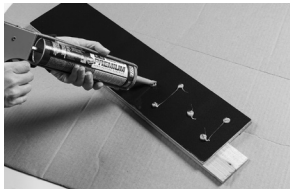
Method 2 - Using high-quality polyurethane construction adhesive.
