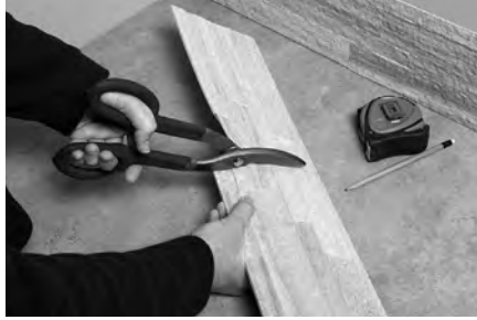
Cutting a straight cut with a snip
