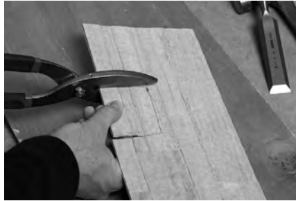
Starting a notch using a snip
