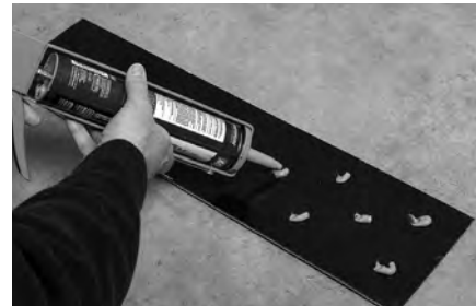
Method 2 - Using high-quality polyurethane construction adhesive
