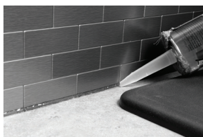
Caulking the counter top seam
