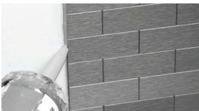
Finishing option 2: Caulking outside edges
