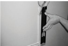
Mark horizontal and vertical reference points
