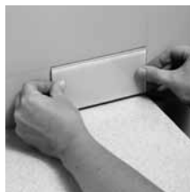
The adhesive on the back of the Aspect Metal tiles is extra sticky and pressure sensitive.
