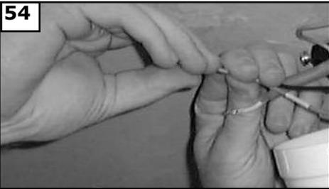
Make wire connections to the power source using wire nuts provided. Make sure that no filaments are outside of the wirenut. After making the wire connections, the wires should be spread apart with the grounded conductor and the equipment-grounding conductor on one side of the outlet box and ungrounded conductor on the other side of the outlet box. Spliced wires should be turned upward and pushed carefully up into the outlet box.
