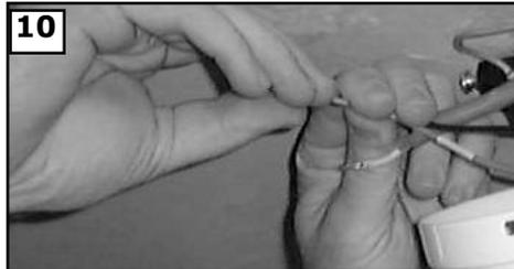
Make wire connections to the power source using wire nuts provided. Make sure that no filaments are outside of the wirenut. After making the wire connections, the wires should be spread apart with the grounded conductor and the equipment-grounding conductor on one side of the outlet box and ungrounded conductor on the other side of the outlet box. Spliced wires should be turned upward and pushed carefully up into the outlet box.
