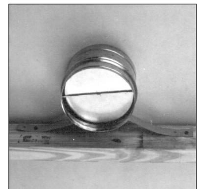
**Step 4** - Snap the grill into the mounting collar. Grill should be pushed tightly into place for an airtight fit.
