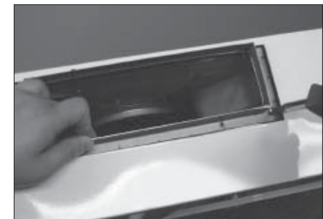
6. Mount starting collar (provided) at rear discharge.
