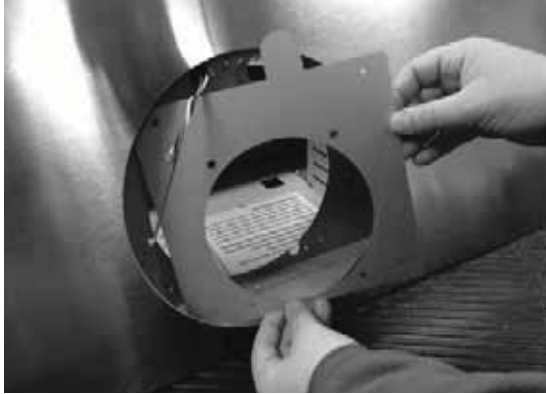
1. Remove internal blower flange plate.
