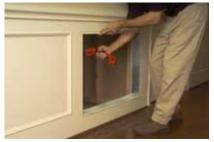
**Step 2. Install Worth metal frame** Insert our metal frame into the prepared opening with the frame flush along the top (side with the spring) of the opening. The side flanges will help ensure a flush mount. Screw the frame into the adjacent wall or ceiling studs.
