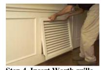
**Step 4. Insert Worth grille** First insert the top of grille with the brackets, just behind the big curl of the frame. TGIF! Ensure brackets are behind the curls on the metal frame.
