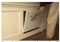
**Step 1. Remove old metal grille** For remodeling, cut around any existing caulking on your old metal grille. Remove its screws or nails, than simply pull out the entire grille assembly from the opening.
