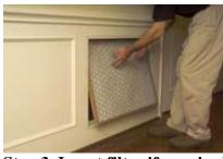
**Step 3. Insert filter if required** If your system requires a filter at the return air grille, insert your filter now. Remember - Top Goes in First (TGIF)!
