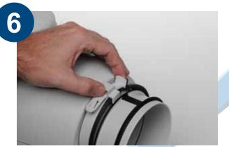
Re-mount fan body by tightening the clamps.
