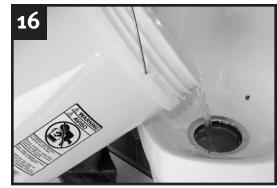
Pour 5 gallons of water as rapidly as possible into housing to ensure good flow and no leaks or standing water.
