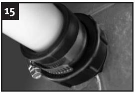
Tighten the compression nut and gear clamp.
