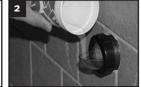
Clean face of existing wall flange then install the 2" compression nut with the clear inspection disc. Slowly pour water into the drain.
