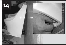
Hang the bowl, inserting tailpipe into bushing, then install anchor screws with washers.
