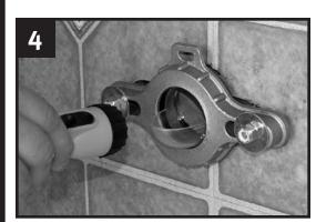
Use a flashlight to check pitch/slope. There should be no water present in the inspection disc or nipple. Remove flange after inspection.
