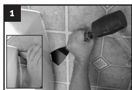
Use utility knife to cut caulk, then use a putty knife and mallet to remove the bowl. Remove hanger brackets, scrape off caulk, and clean the wall.
