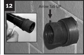
Apply lubricant to the outside of the rubber bushing and ribbed inside area. Insert the tube and bushing with the arrow tab at the top.
