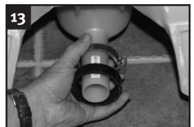
Place the gear clamp and compression nut onto the housing tailpipe. Apply lubricant to the tailpipe.
