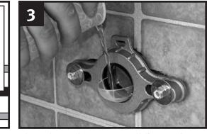
Clean face of existing wall flange then install the brass flange with the clear inspection disc. Slowly pour water into the drain.
