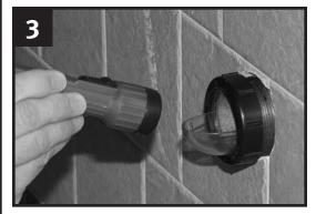
Use a flashlight to check pitch/slope. There should be no water present in the inspection disc or nipple. Remove compression nut after inspection.
