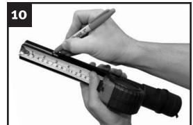
Find the drain nipple depth on the cutting chart (left) and mark the specified trim length on the insert tube at the nearest 1/4" groove.
