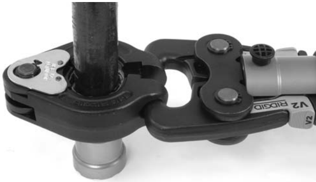
Figure 11A – Placing V2 Actuator Tips Into MegaPress Ring Pockets
