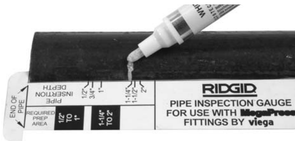
Figure 6B – Marking the Pipe Before Inserting Into Fitting Using RIDGID® MegaPress® Pipe Inspection Gauge
