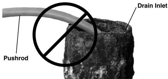
Figure 18 – Avoid Pulling At Sharp Angles
