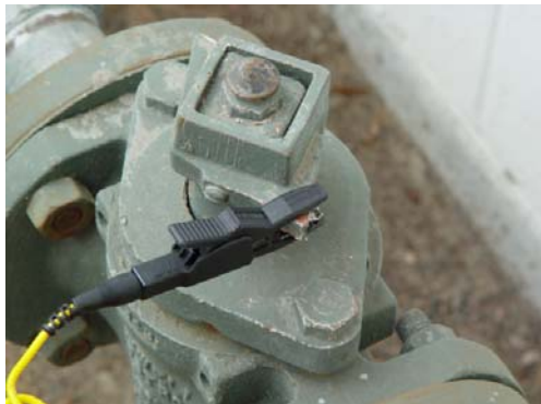
Figure 8: Example of Connecting to a Gas Line
