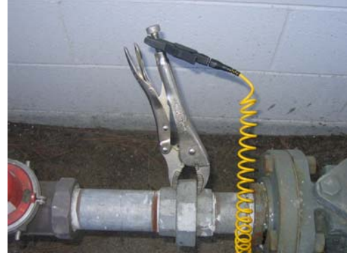
Figure 9: Alternative Connection to a Pipeline
