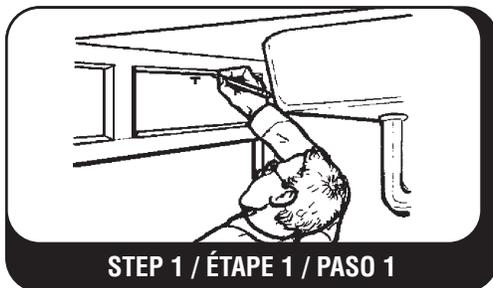
Using a sharp soft lead pencil (so you can erase later), trace the frame perimeter on the false front panel inside. Mark a small "T" for top panel reference.
