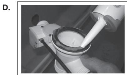
7. Apply 1/8" continuous bead of 100% silicone sealant to back side to metal strainer as shown in photo **E**. Press Strainer retaining bolt into metal strainer and insert into drain hole of acrylic bath.
