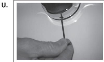
21. Rotate left and right lightly to feel stops in drain cable control. This opens and closes drain.
