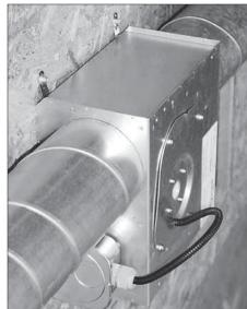
The 'LPK'-fan can easily be mounted with the four brackets in any position.
