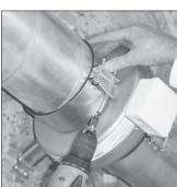
3. Strap the duct clamps on each side of the fan with the screws.
