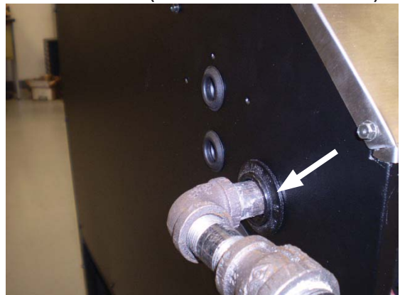
FIGURE 28 - FURNACE GAS PIPE CONNECTIONS (NOTE RUBBER GROMMET)
