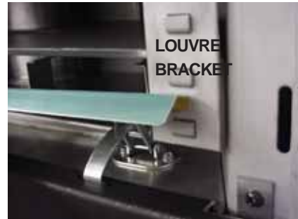
FIGURE 37 UPPER LOUVRE INSTALLATION
