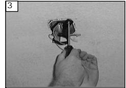
Install the Mountiing Bracket to the Outlet box. Use only the screws provided with the outlet box.
