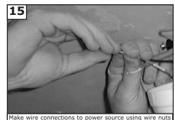
provided. Make sure that no filiments are outside of the wirenut. After making the wire connections, the wires should be spread apart with the grounded conductor and the equipment-grounding conductor on one side of the outlet box and ungrounded conductor on the other side of the outlet box.
