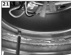
Loosen the pre installed screws of switch housing plate.
