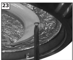
Install 3 screws to install light pan.
