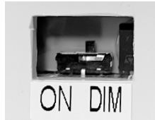
Left side of wall control
